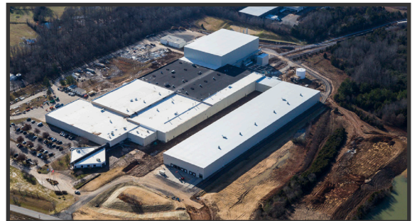
Daltile Campus Expansion | Dickson, TN 496,283 Square Feet
