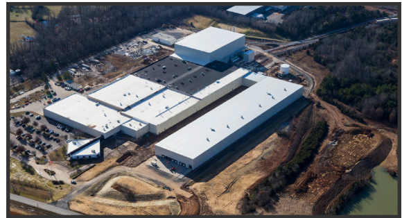
Daltile Campus Expansion | Dickson, TN 496,283 Square Feet
